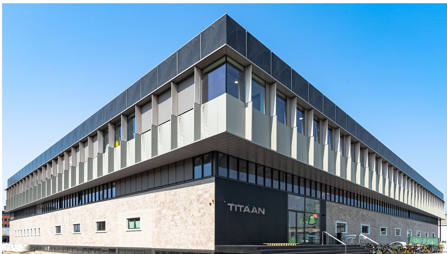
Titaan, The Hague. Patterned solar panels integrated into the upper facade.
