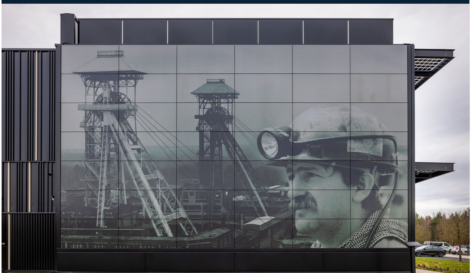
Soltech, Genk. A photographic image printed across a solar facade.
